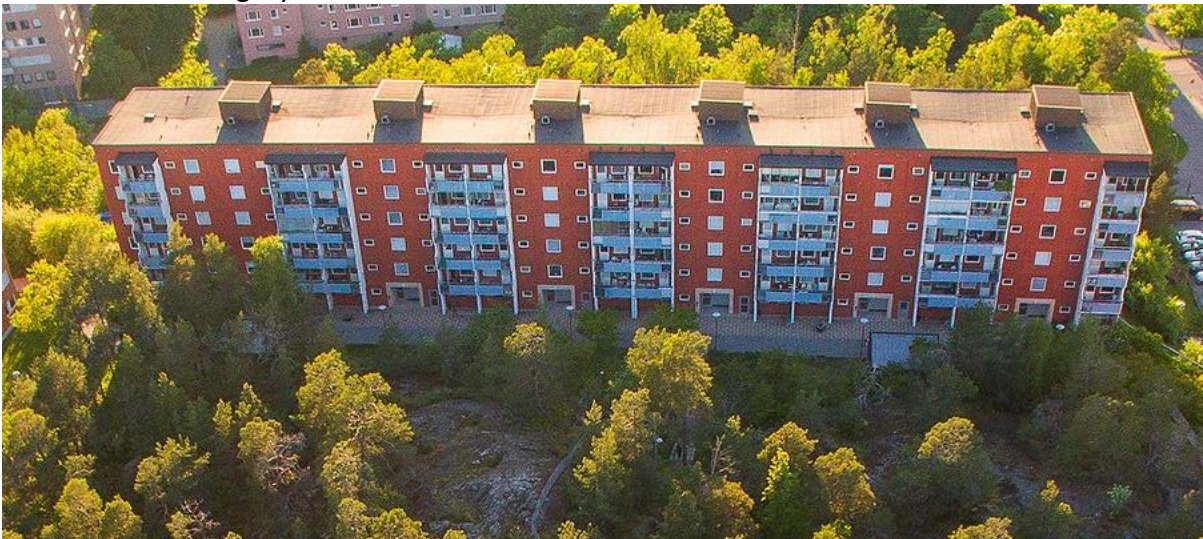
Second Stavangeryard, Stavangergatan 4-16
