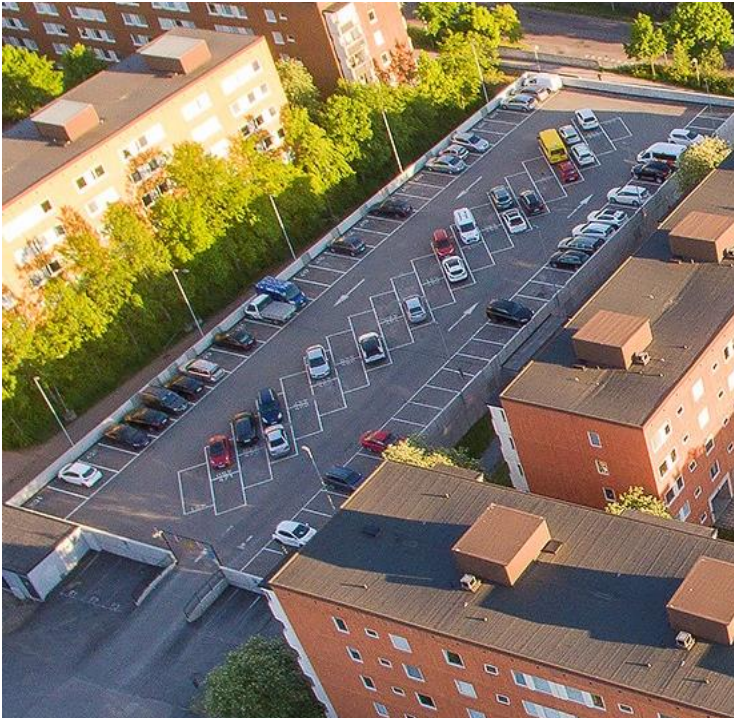
Lofotengatan 1-5, garage on two levels and roof parking
