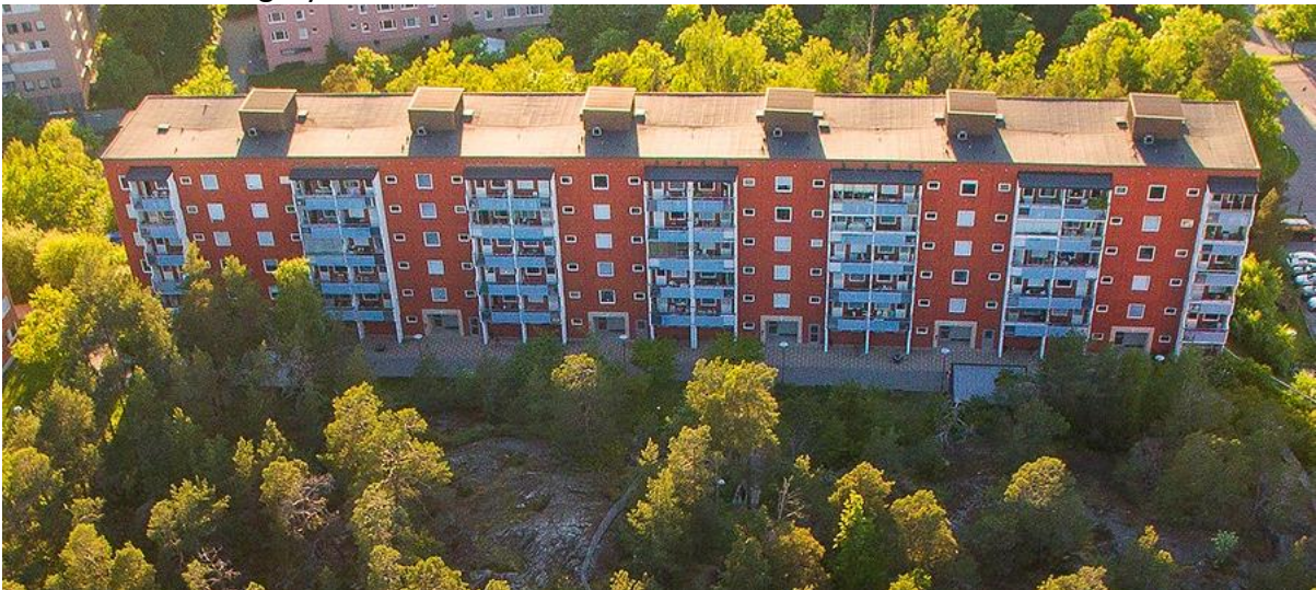
Second Stavangeryard, Stavangergatan 4-16
