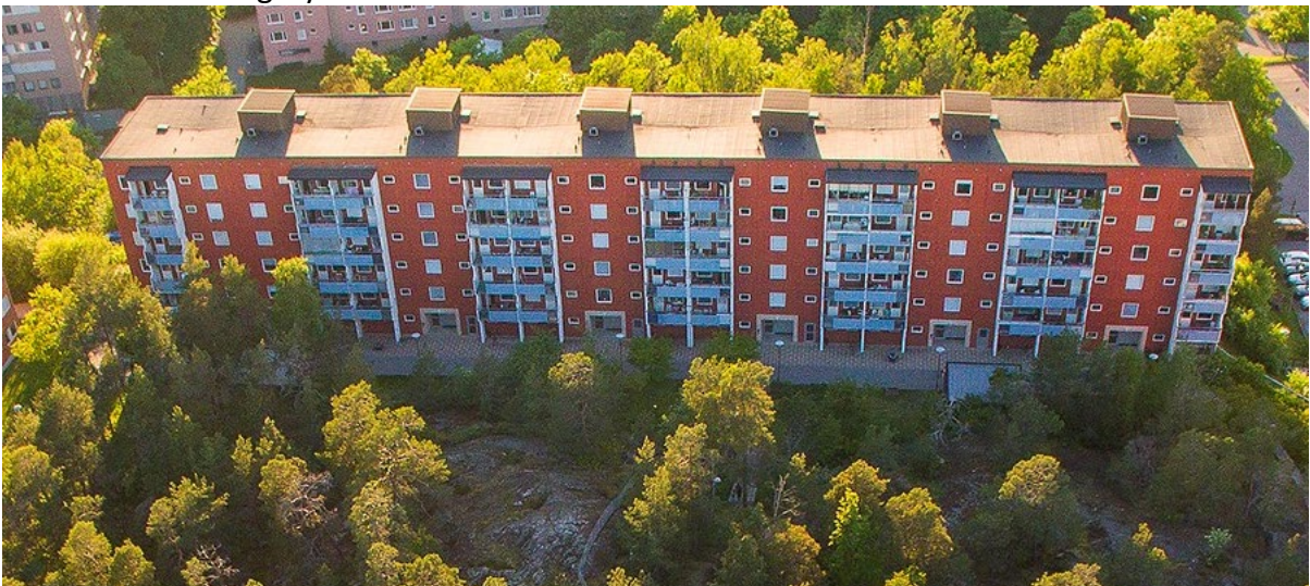
Second Stavangeryard, Stavangergatan 4-16
