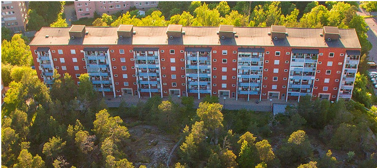
Second Stavangeryard, Stavangergatan 4-16
