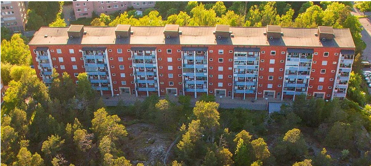
Second Stavangeryard, Stavangergatan 4-16
